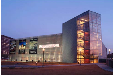
Denver Art Museum Parking Structure Source: Mortenson
