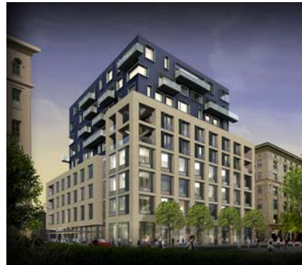
Sugar Building at 16 th & Blake from Denver Infill.com
